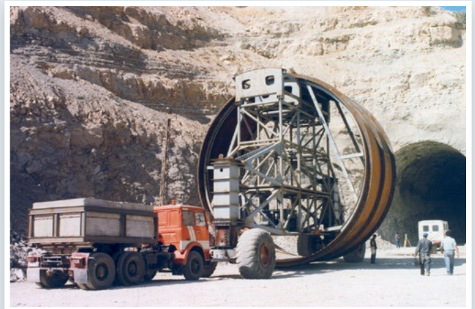
Tunnel Steel Lining (During Erection)
