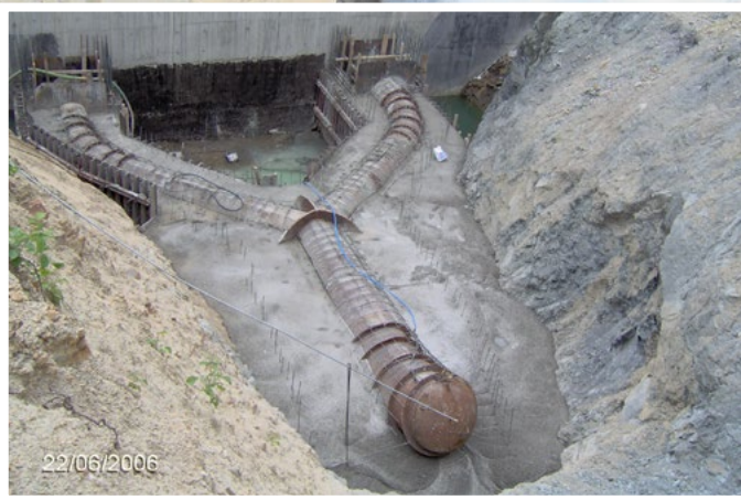
Bifurcation Pipe (Under Pressure Test)
