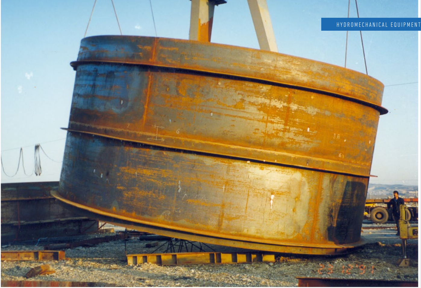
Penstock Fabrication at site and prefabrication Area. Total= 35 tons.
