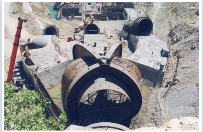
Trifurcation Branch Pipe (During Erection)
