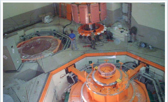
Turbine Erection
