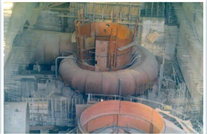
Spiral Case and Stay Ring, During Erection
