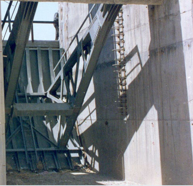
Radial Gates for Irrigation Regulator
