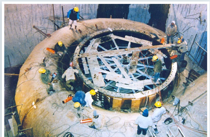
Spiral Case and Stay Ring During Erection
