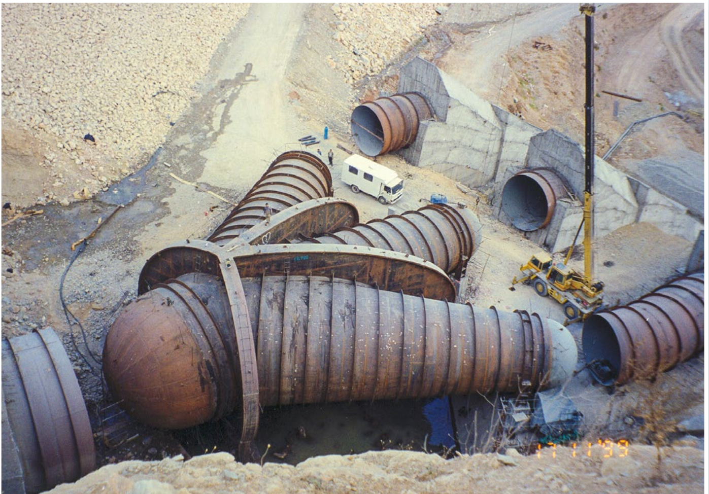
Trifurcation Branch Pipe, \varnothing inlet= 9500 mm / \varnothing outlet= 5000 mm x 3 / Weight= 700 ton
